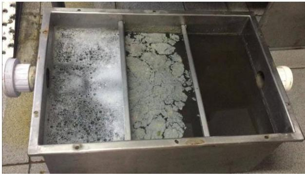
Portable grease trap is cleanup only twice a week using EM
